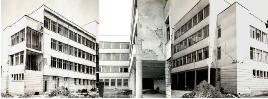
Figure 7: School in Strazhitza (1986) – Complex Configuration and Absence of Seismic Joints.
